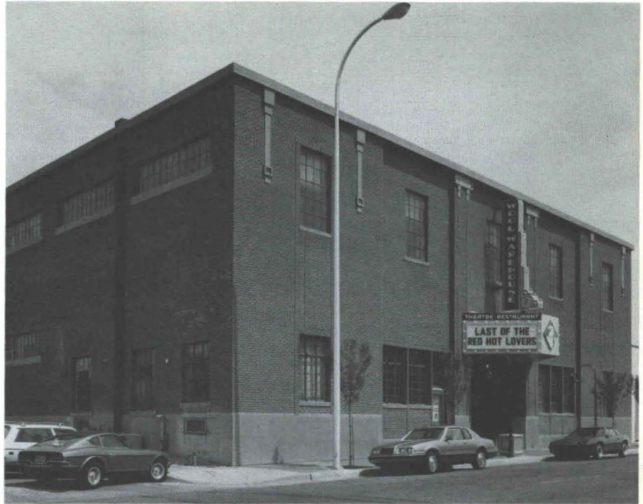
Figure 4 — Exterior view of the wool warehouse.
